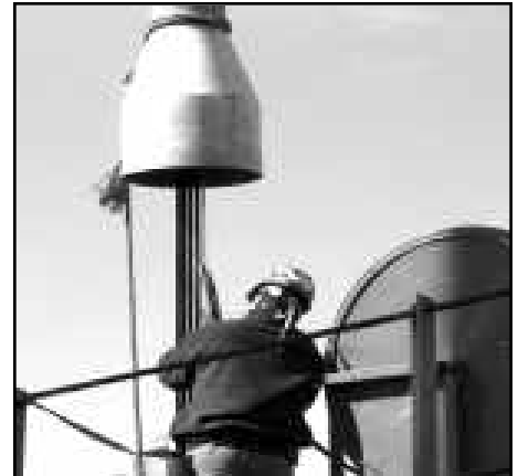
Above: After the master cable is anchored, it takes a couple of days to thread the rest of the steel cable strands through the pipe and into the anchorages.
